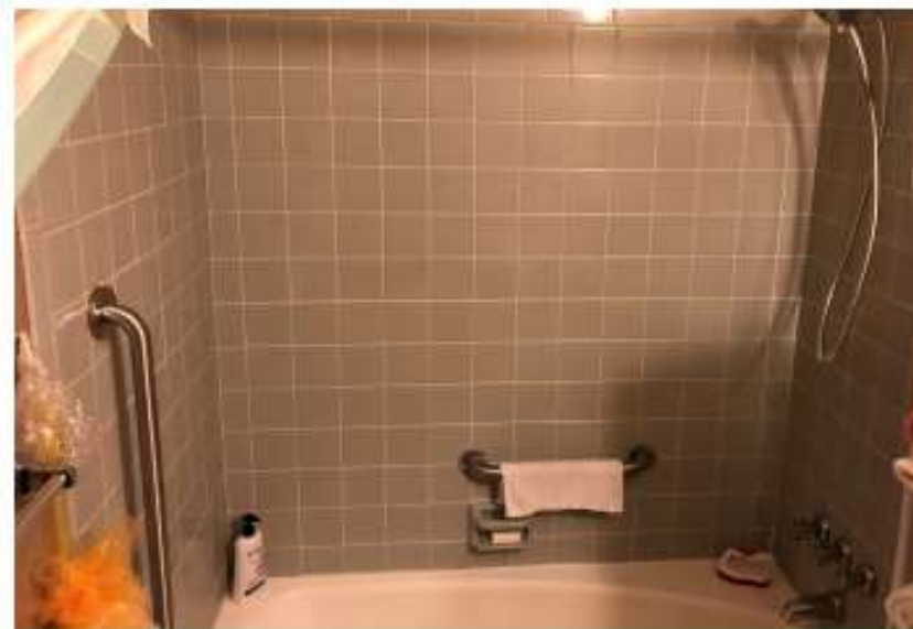
shower grab bars and handheld shower head
