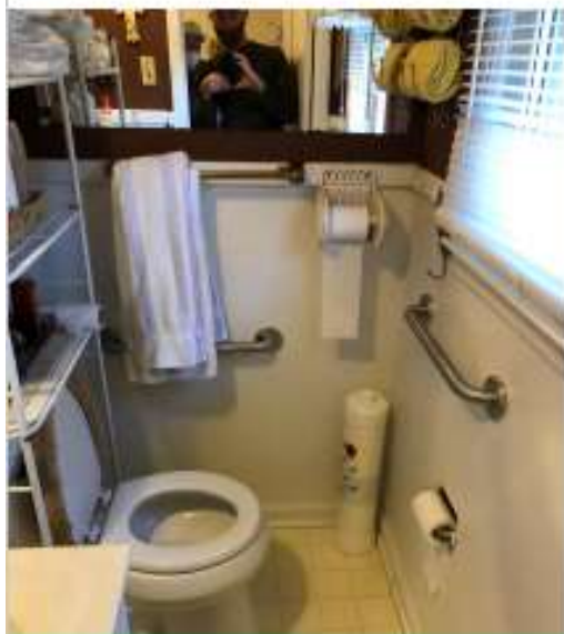
grab bars next to toilet
